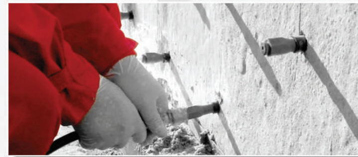
Concrete Injection
