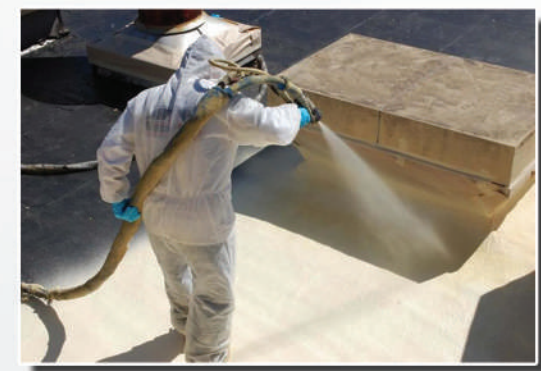
Spray Polyurethane Foam Roofing
