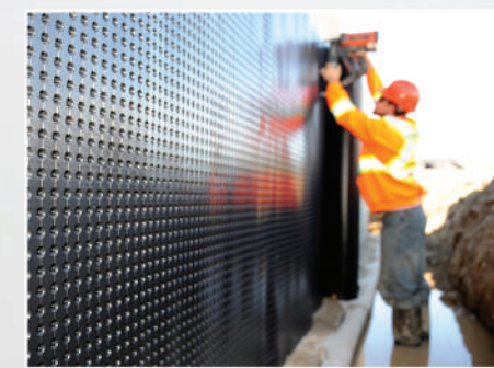
Waterproofing Membrane Application (PVC - TPO - HDPE)
