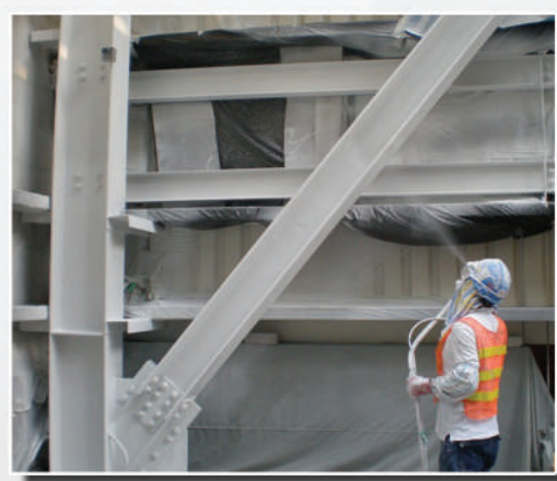
Intumescent paint application
